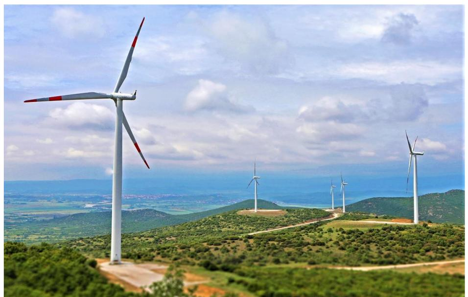
Bogdanci Windpark. The WBIF funded the feasibility study and the impact assessment for the park from a €400,000 EU grant. The first phase of the project is already in operation, 16 turbines of 36.8 MW, while the capacity of the windfarm is currently being increased to 50 MW.
