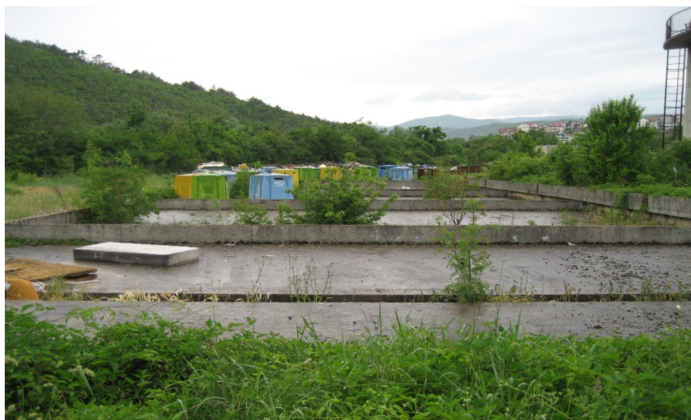
Existing wastewater infrastructure in Široki Brijeg, after several years of disuse (to be rehabilitated).
