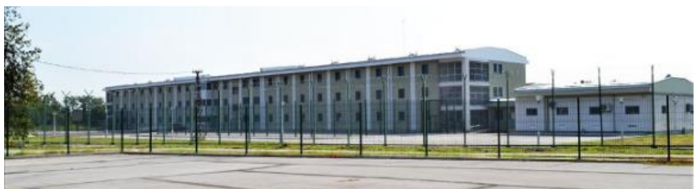
Idrizovo PCF – Semi-Open Section Exterior
