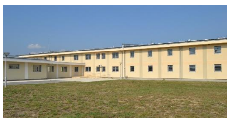
Idrizovo PCF – Open Section Exterior
